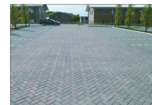
Priora Permeable Paving
