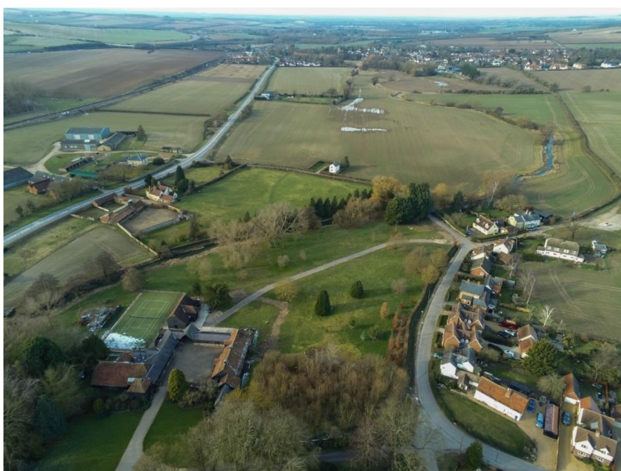
Figure 2.9 Aerial view of River Cam and flood zone between Little Chesterford and Great Chesterford
