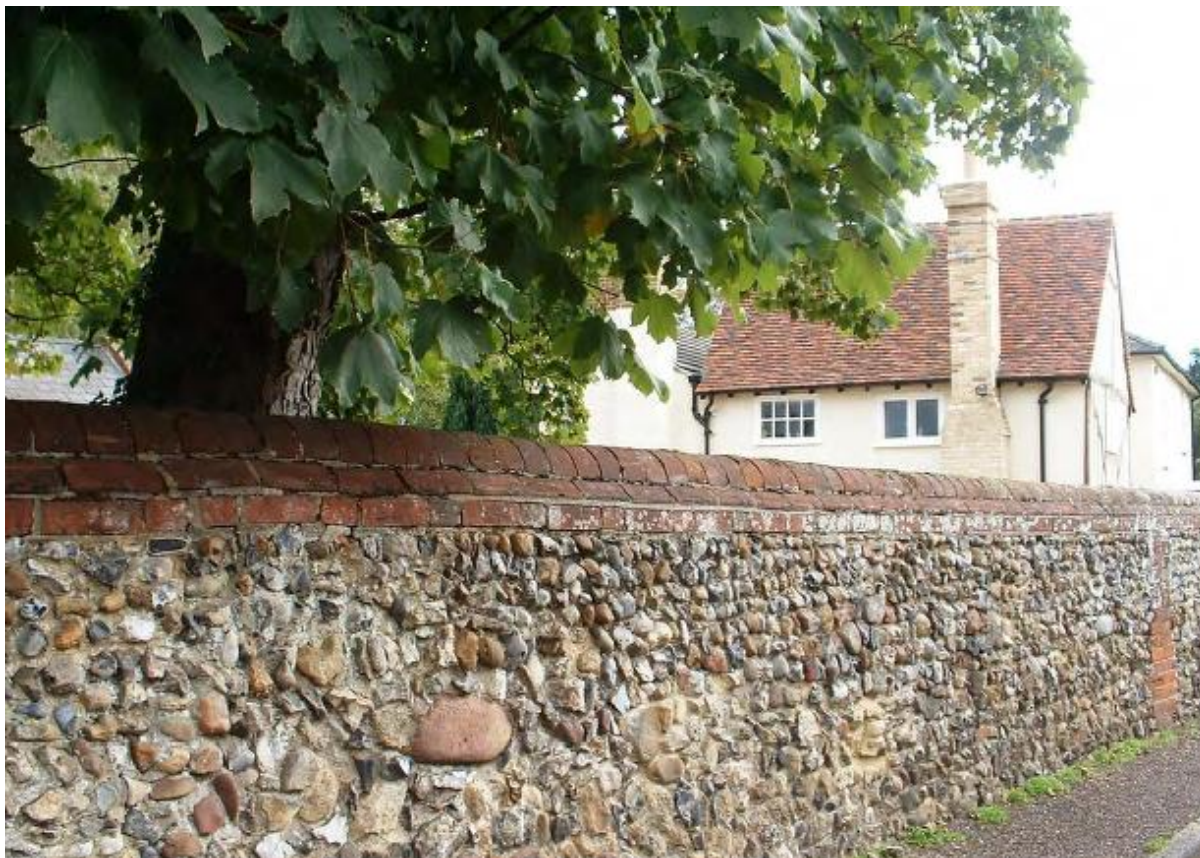
Photo 9 – Brick and flint wall at Carmen Street
