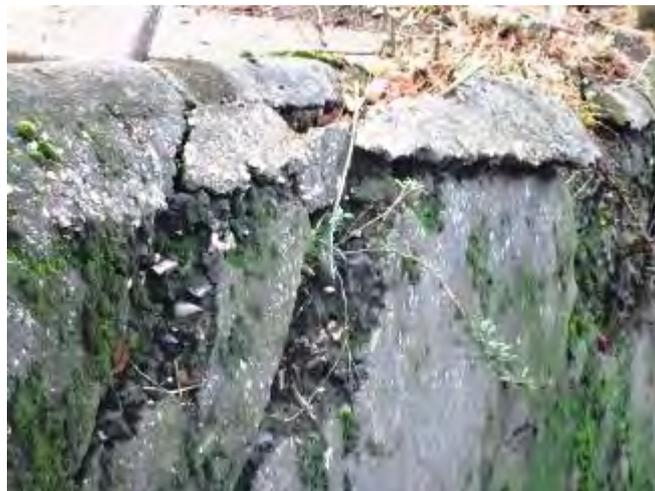
Decayed area of black concrete wall in poor repair at west side of Thaxted road
