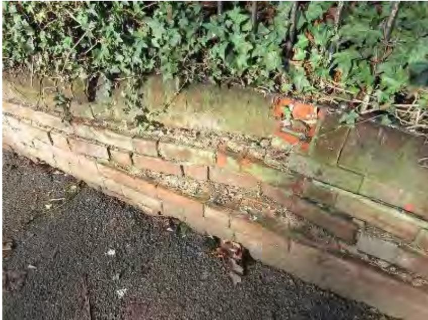
The damaged brickwork under the railings near to the Thaxted Road/Chaters Hill traffic lights
