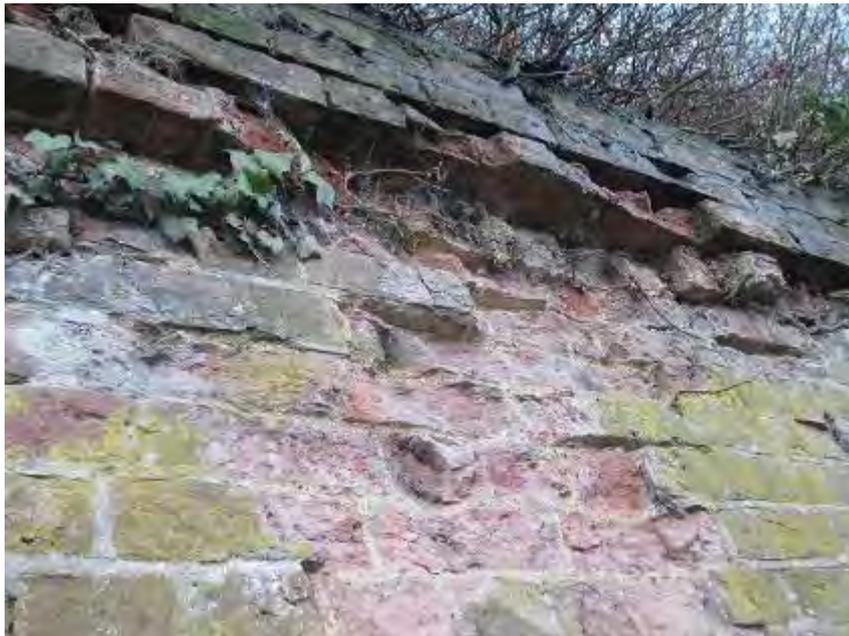
The poor condition of the old railway bridge retaining wall brickwork.
